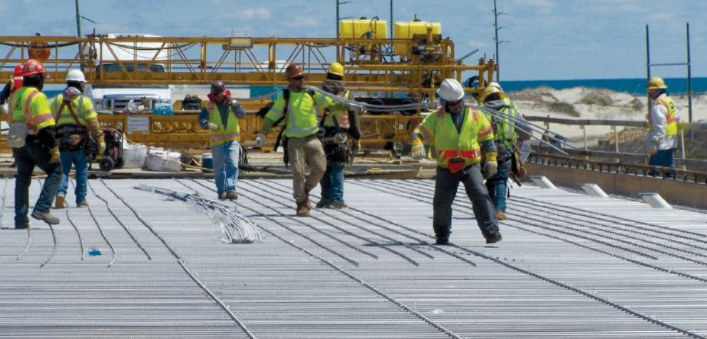
The Marc Basnight Bridge is designed to resist corrosion in the harsh saltwater environment of coastal North Carolina. To meet the 100-year service life, the design team chose stainless steel reinforcement for the cast-in-place concrete deck.
