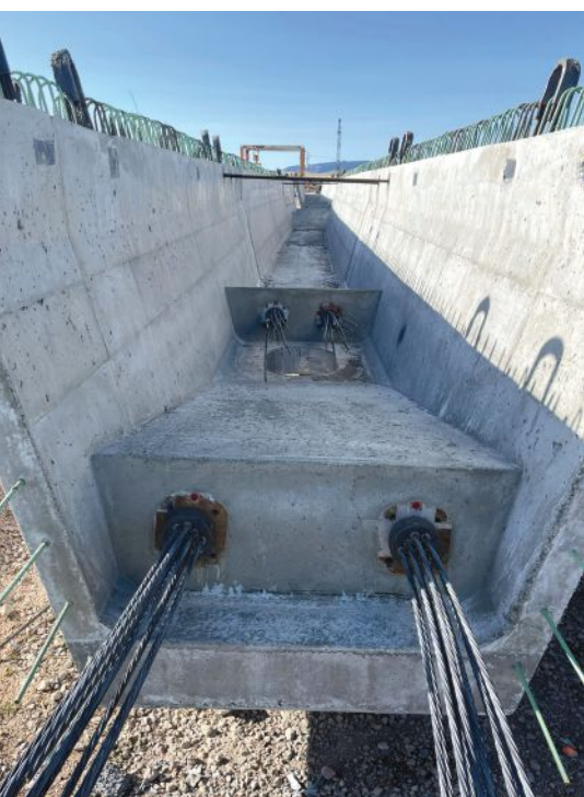
The simple-made-continuous design uses precast, post-tensioned concrete tub girders in a manner similar to that used for pretensioned girders. The girders were tensioned in the casting yard after they were removed from the forms, but before they were shipped.
