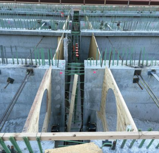
Temporary and permanent bracing is in place as the formwork and reinforcement for the continuity diaphragms at the piers are prepared.
