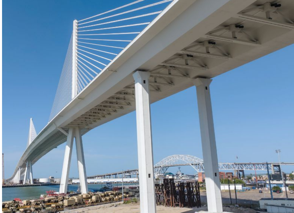
Underside view of twin box girders and delta frames.
