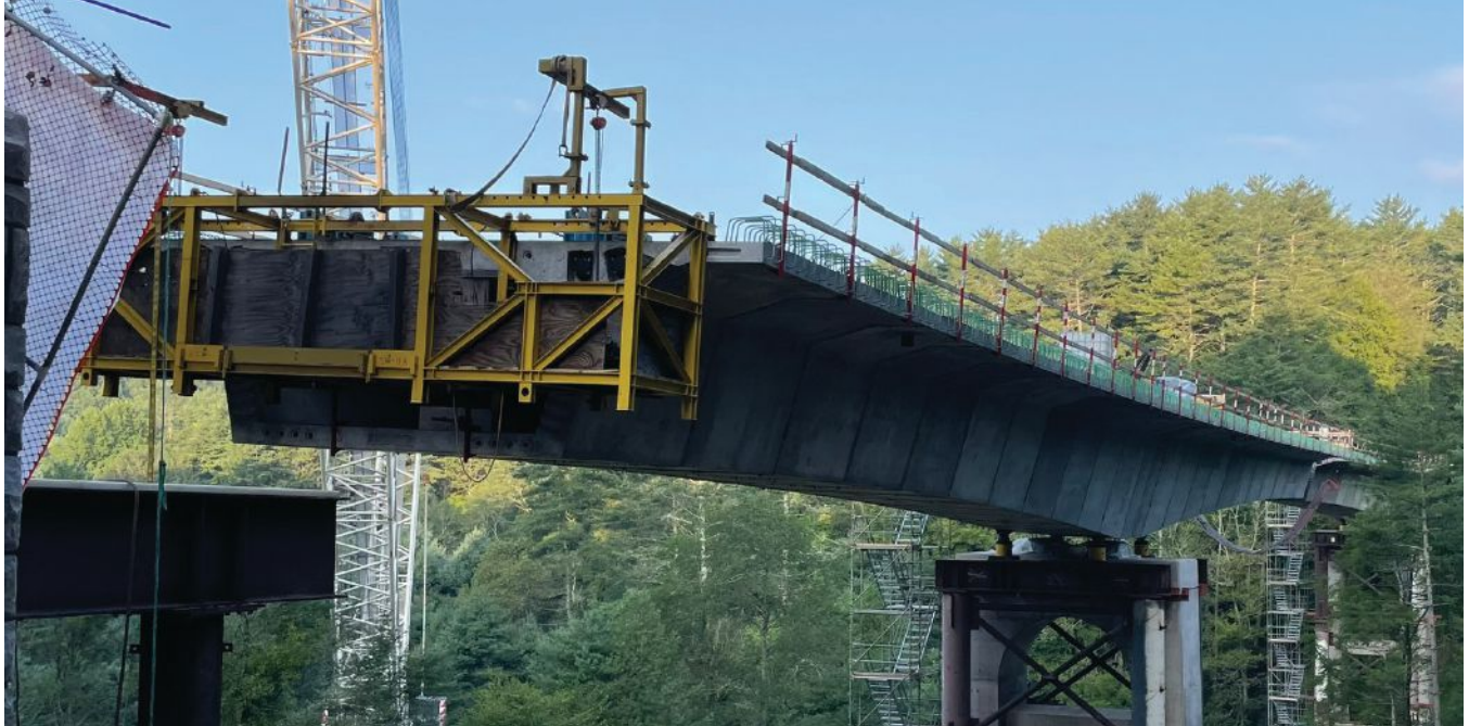
During construction, before the closure pour, the cantilever is supported by temporary towers. Photo: COWI North America.
