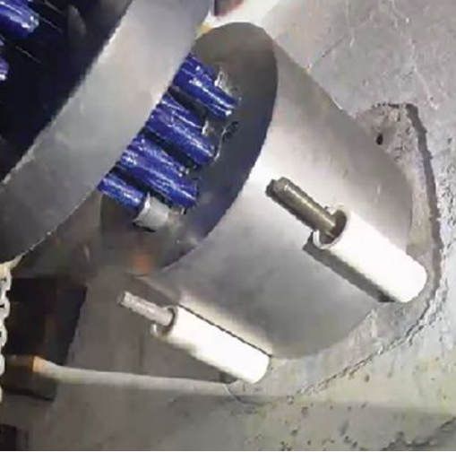
Anchorage of an unducted continuity tendon. Photo: Vannoy Construction.
