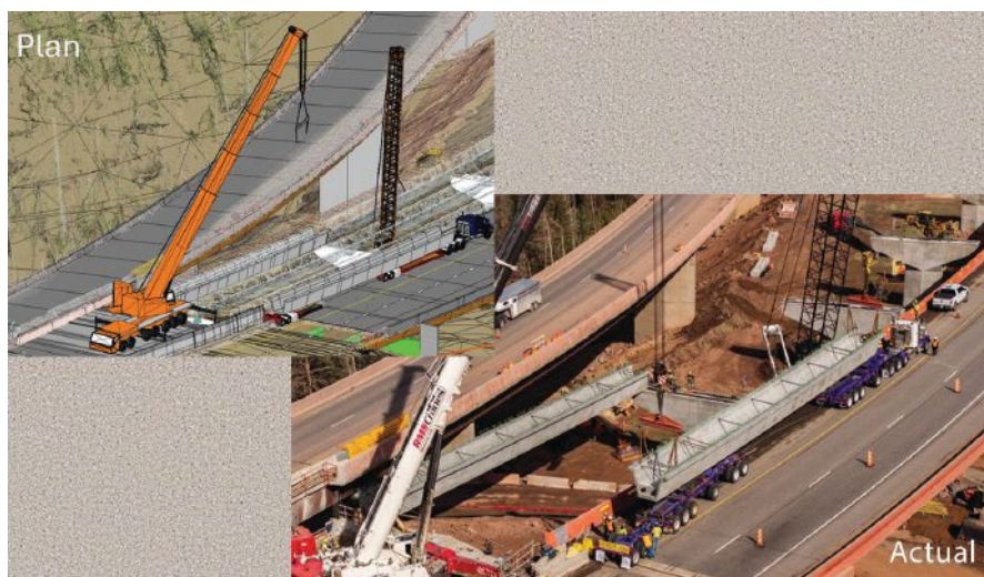
Linking three-dimensional models (upper left) to construction timelines can help with scheduling, construction staging, and the like. Figure: Kiewit/Bentley Systems.
