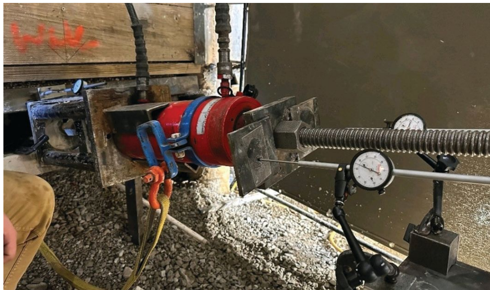
A post-tensioned bar being tensioned in the field. Photo: Pete Speier, Williams Form.
