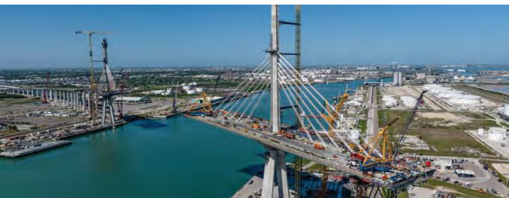
Construction of the new Harbor Bridge tower and superstructure.
