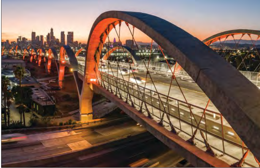
The Los Angeles Bureau of Engineering's Sixth Street Viaduct is a cast-in-place concrete network tied arch that sets a new threshold for seismic safety and expands the utility of urban bridges. Photo: ACI Excellence in Concrete Construction Awards.
