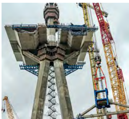
A delta frame is installed using a custom support system.
