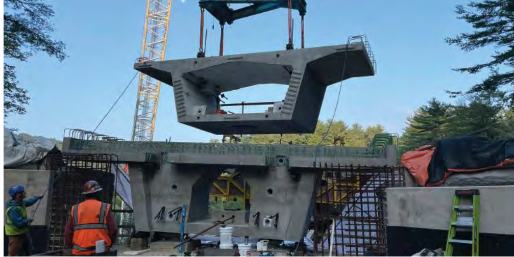
A revised precast concrete box-girder segment is lifted during erection. Photo: COWI North America.
