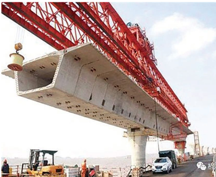
Figure 1. A concrete segmental bridge structure is constructed using precast concrete segments. Figure: Datai Crane.
