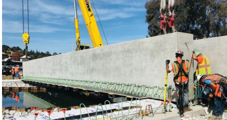
A tandem crane pick is used to place a 154-kip mainline track edge girder on the abutments.
