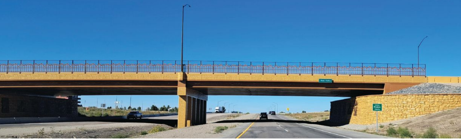
Figure 4. The completed Fort Hall Interchange project features a 222-ft-long, 88-ft-wide bridge spanning Interstate 15 in Fort Hall, Idaho, with newly developed elements crucial for its location in a high-seismic region.
