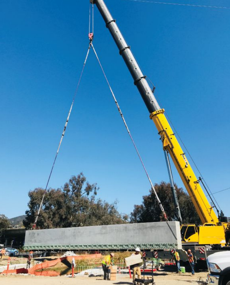
A tandem crane pick is used to place a 154-kip mainline track edge girder on the abutments.
