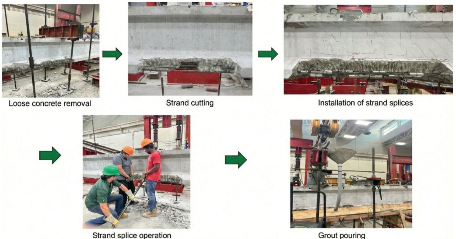
Figure 6. After the girders were impact tested, these steps were taken in the strand splicing repair.
