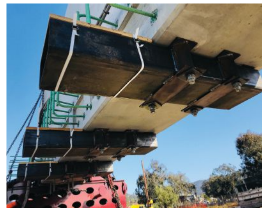
View from beneath an edge girder. No falsework was permitted in the creek, so the team developed a temporary support system to support the floor beams during construction. The supports were later repurposed to facilitate installation of the bridge's transverse post-tensioning. All Photos: Stacy Witbeck/Herzog.
