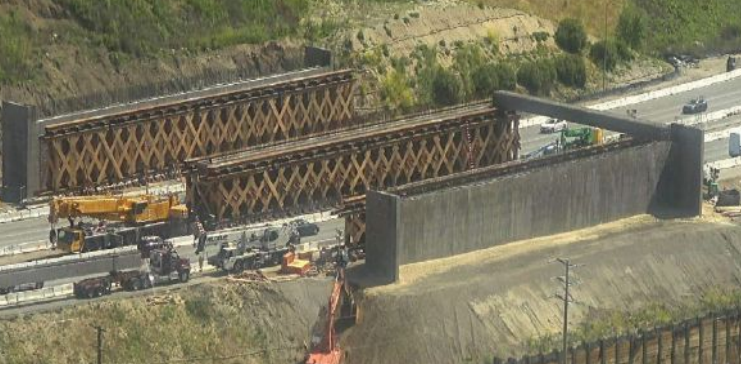
The first precast concrete girder is placed. Shoring is used for girder support until the bent caps and girders are connected through the cast-in-place concrete keys and placements. Photo: California Department of Transportation.
