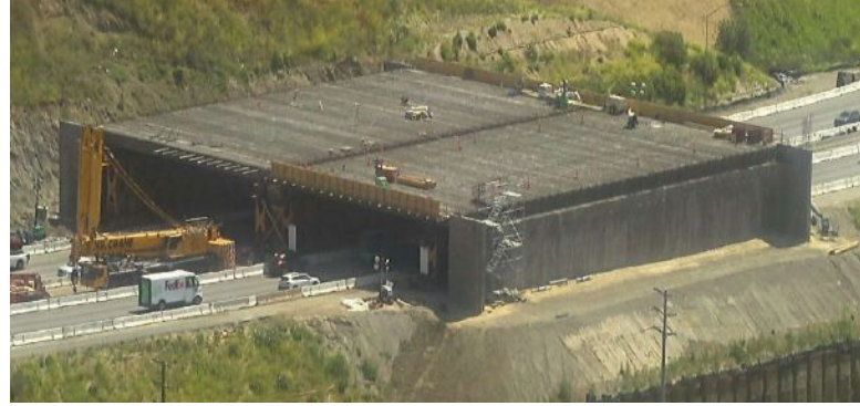
Construction on the precast concrete girders continues. Photo: California Department of Transportation.
