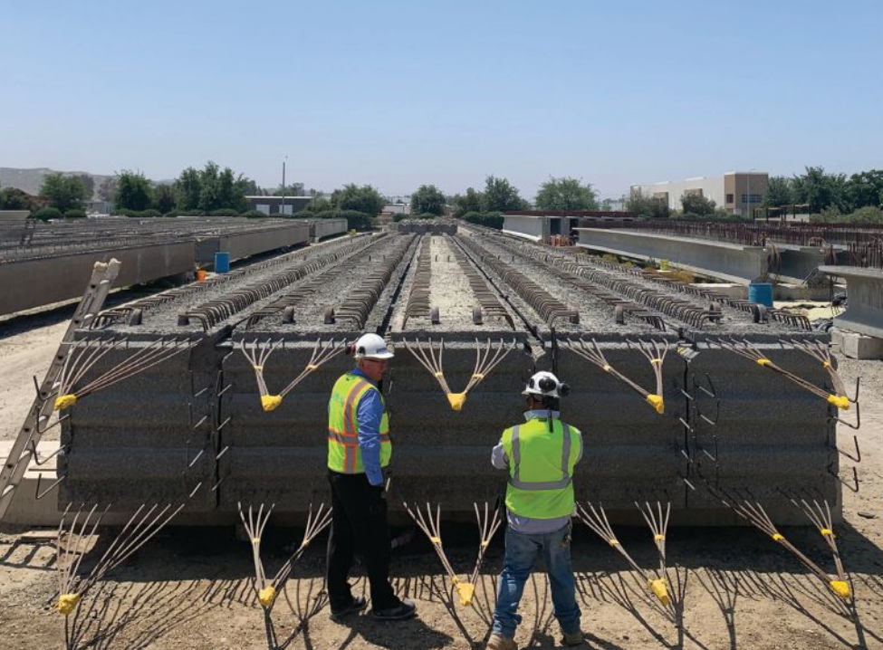
Precast concrete girders in the precast concrete manufacturer's yard. Photo: Coreslab Structures.
