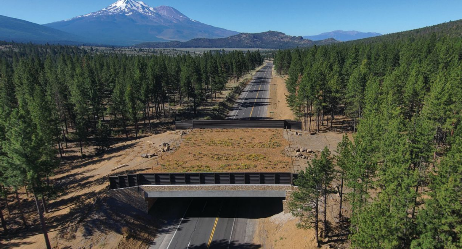
Finished in 2025, the Grass Lake Wildlife Overcrossing provides safe passage for many animals across U.S. Route 97 in northern California. Photo: California Department of Transportation.
