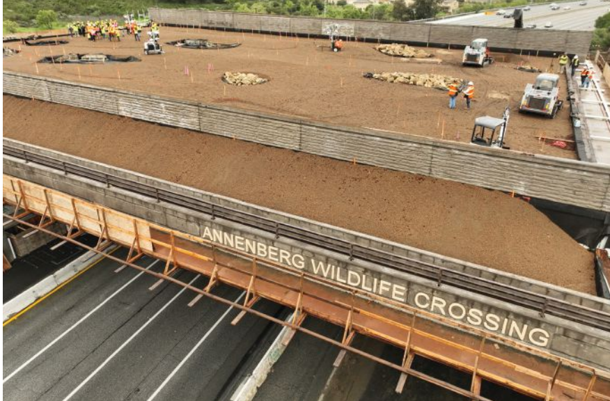
The central deck area serves as natural habitat for wildlife crossing, and each side is bordered by an 11-ft-tall sound wall and vegetated buffer landscape. Photo: Rock Design Associates and National Wildlife Federation.
