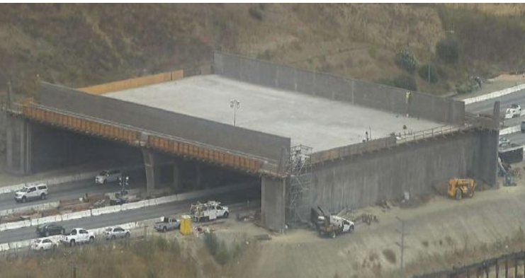
Construction of the cast-in-place concrete sound wall. Photo: California Department of Transportation.
