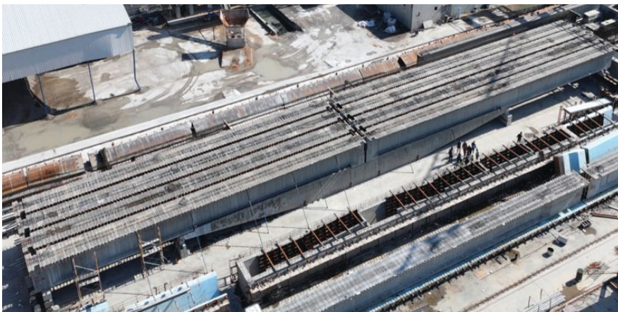
Figure 5. Trial fit-up at the precast concrete producer's yard using actual I-girder and haunch segments.
