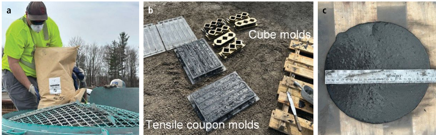
Figure 4. Field-mixing process: (a) Worker loads steel fiber into IMER-750 mixer; (b) molds for making specimens in the field; (c) flow testing to ensure viability of the ultra-high-performance concrete mixtures.
