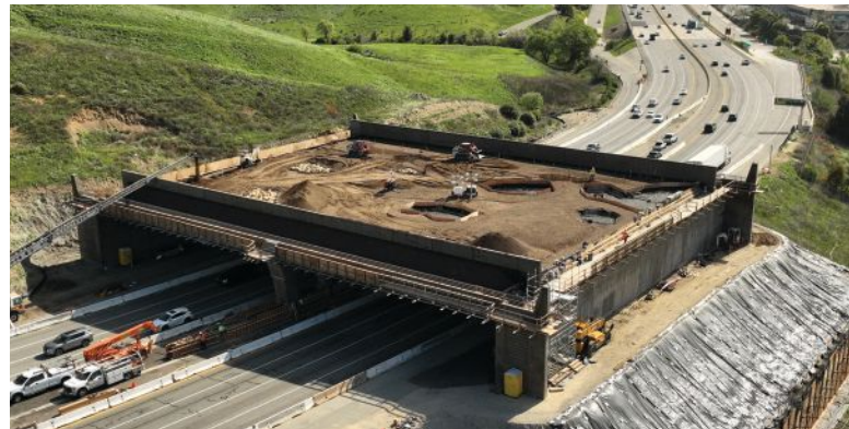
Between 1 and 4 ft of engineered soil creates artificial topography, provides drainage, and supports native vegetation. Photo: California Department of Transportation.
