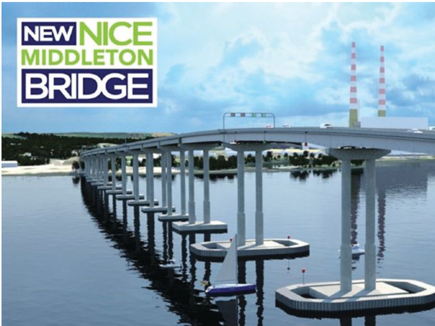
The 1.7-mile, four-lane Harry Nice Middleton Bridge connecting Maryland and Virginia over the Potomac River has a 100-year service life due in part to a corrosion protection plan developed by Siva Corrosion Services.
