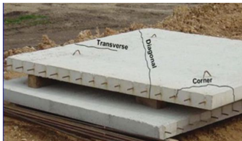
One of the anticipated topics in the CBEI Bridge Deck Construction Inspection course is the on-site inspection of precast concrete deck panels. Shown here are illustrations of types of cracks that may appear after the initial fabrication inspection. Photos: Texas Department of Transportation.
