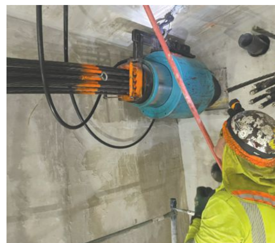
Tensioning the strands of a post-tensioning (PT) tendon. One advantage of the design-build delivery for this project was that the post-tensioning (PT) material supplier was chosen and engaged during the initial design phase. They worked with the design team as the bridge superstructure design was advanced. Photo: Kiewit.
