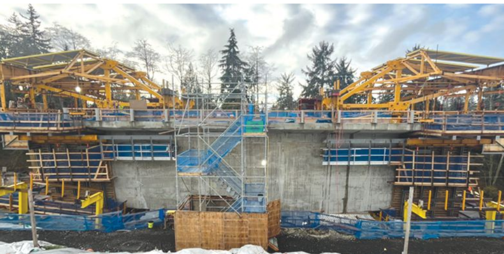
Segments are being cast on both sides of one of the piers. Using four identical form travelers allowed segments to be cast on both sides of both cantilevers concurrently. Photo: Kiewit.
