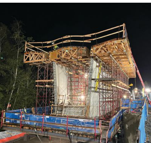
Integrated shop drawings and three-dimensional modeling allowed the design team to spot conflicts before they happened, which was critical to the successful installation of the many reinforcing elements required in the superstructure. Photo: Kiewit.
