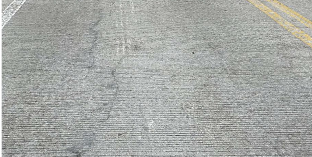
An example of longitudinal cracking in a concrete bridge deck.
