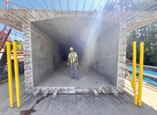
Cast-in-place concrete box-girder segments vary in height from 12.5 ft at the midspan to 25 ft at the piers and typically have a width of 28 ft 9 in. The bottom-slab post-tensioning ducts and web shear keys are visible. Photo: Kiewit.
