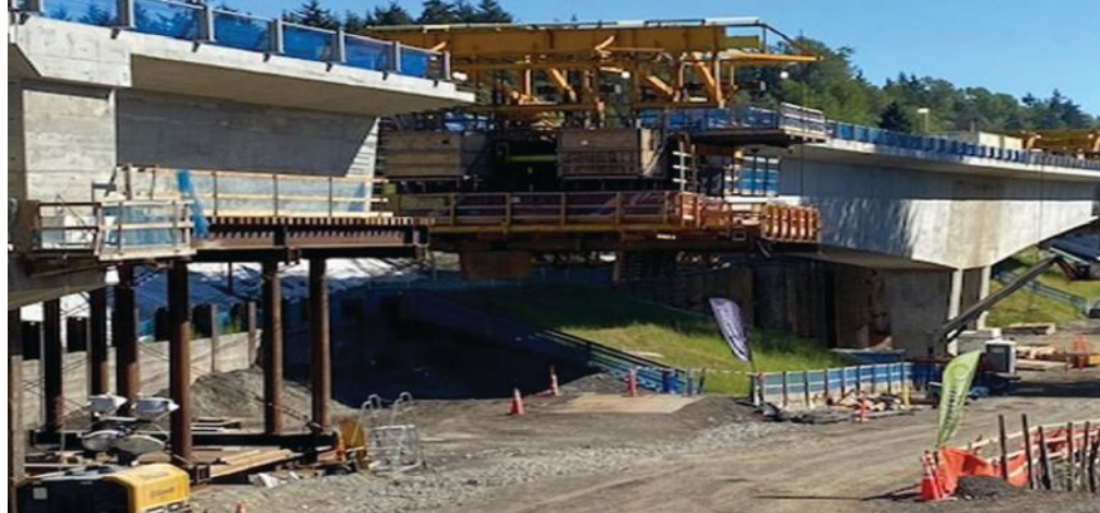
Two sections of the back spans were cast on falsework at either end of the structure for a length of about 50 ft, while the remainder of the segmental structure was constructed using form travelers and the balanced-cantilever construction method. Photo: Kiewit.
