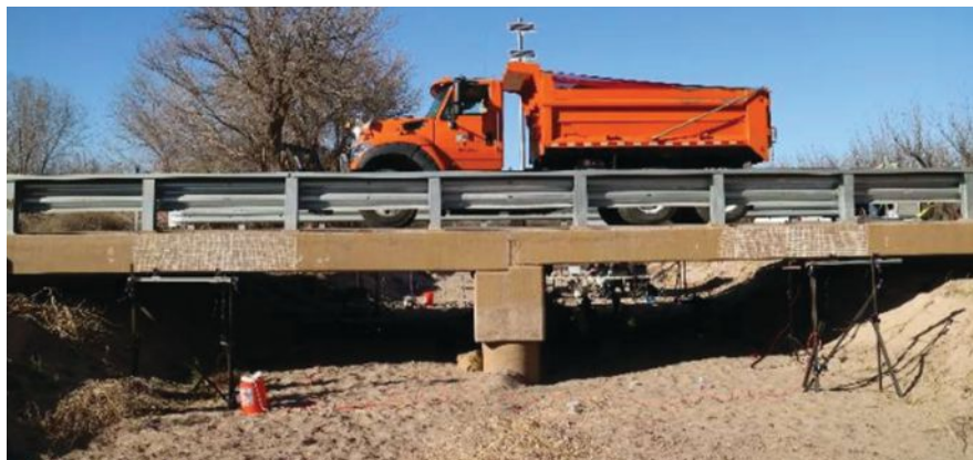
Figure 5. Load testing on the NM 186 over La Union Main Canal. This is the New Mexico Department of Transportation's first use of ultra-high-performance concrete (UHPC) for a prestressed concrete girder bridge. One span of the two-span bridge used UHPC, and the other span used a conventional concrete mixture. Photo: New Mexico Department of Transportation.
