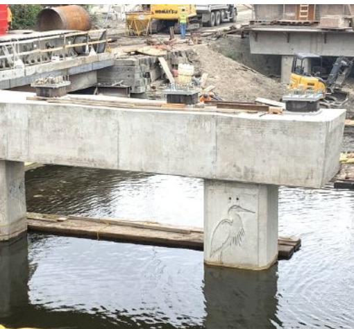
Seismic isolation bearings—rubber bearings with lead cores—reduce the seismic demand on the concrete columns and foundation. Great blue herons are featured on the pier columns because the Sammamish River is a major habitat for the species. Photo: Jacobs.
