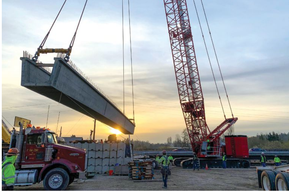
Installing one of the precast, prestressed concrete tub girders. The typical girder is 110 ft long and weighs 165 kip. Photo: Jacobs.
