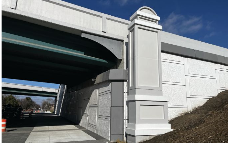
A component of the project's aesthetics and enhancements implementation plan is the placement of precast concrete corner monuments ranging from 22 to 38 ft in height. Here, a decorative monument is located adjacent to mechanically stabilized earth abutment walls. Photo: Janssen & Spaans Engineering.
