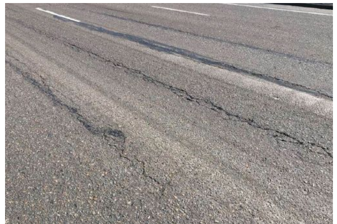
Figure 1. Examples of side-by-side precast, prestressed concrete slab bridges with keyway failures. On the left is a broken, full-width tie rod hanging from the side of a prestressed concrete slab. The photo on the right shows reflective cracks at the joints between prestressed concrete slabs. All Photos and Figures: Oregon Department of Transportation.
