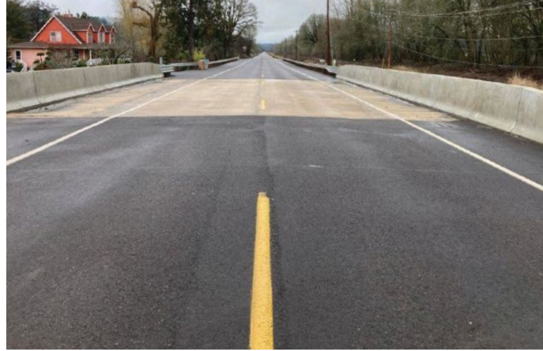
Figure 6. The West Fork Dairy Creek Bridge after installation of a ¾-in.-thick polymer concrete overlay.
