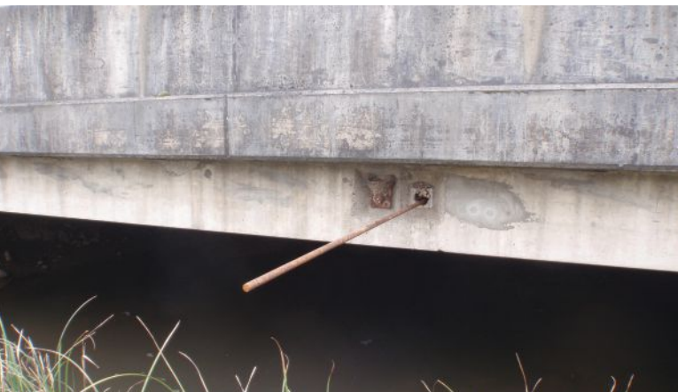
Figure 1. Examples of side-by-side precast, prestressed concrete slab bridges with keyway failures. On the left is a broken, full-width tie rod hanging from the side of a prestressed concrete slab. The photo on the right shows reflective cracks at the joints between prestressed concrete slabs. All Photos and Figures: Oregon Department of Transportation.
