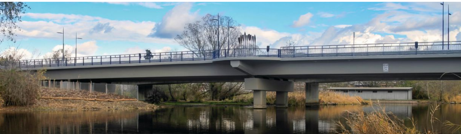
Nine vertical “oars” at the overlook on the West Sammamish River Bridge multiuse path delineate its position and importance Photo: Jacobs.
