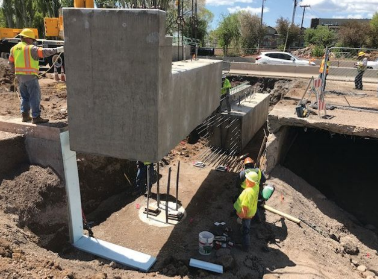
The Rio de Flag Bridge in Flagstaff was replaced in less than a week using accelerated bridge construction methods like prefabricated box beams and precast concrete abutment caps. Photo: NFra Inc.
