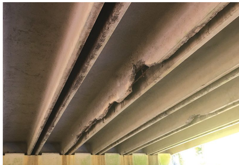
Figure 1. The C-channel bridge in Sampson County, N.C., which was closed to traffic in May 2020, exhibits typical deterioration experienced by C-channel beams. All Figures: North Carolina State University.
