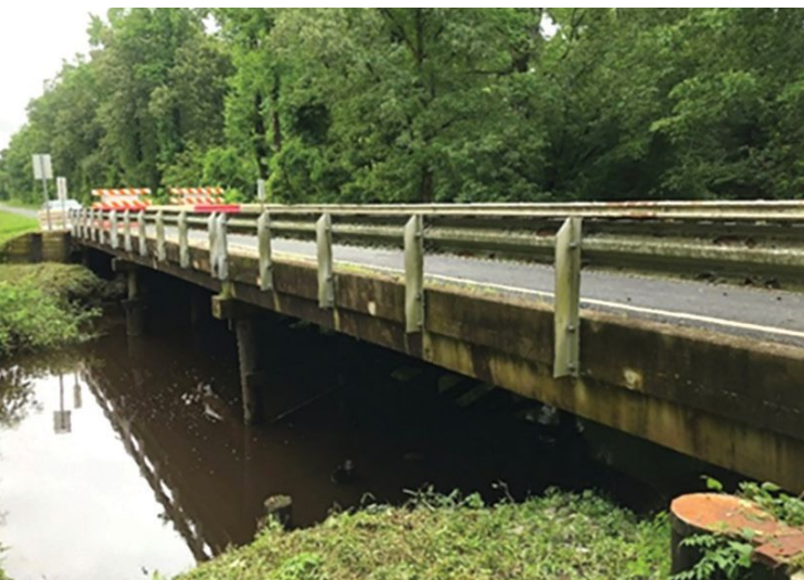
Figure 1. The C-channel bridge in Sampson County, N.C., which was closed to traffic in May 2020, exhibits typical deterioration experienced by C-channel beams. All Figures: North Carolina State University.
