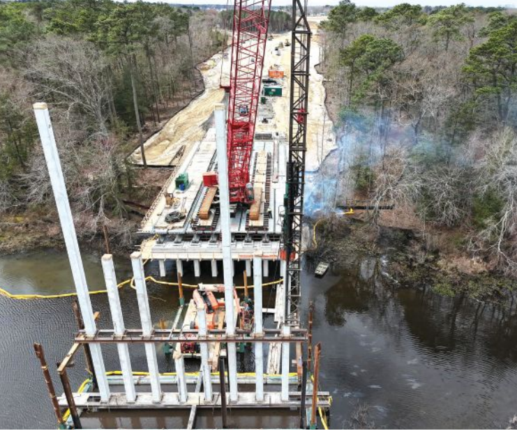
Figure 2. A crawler crane is used to erect Bridge 596 of the Millsboro Bypass project in Sussex County, Del. The engineer of record and the specialty engineer collaborated to ensure that the bridge design accounted for the construction loads. Photo: Richard E. Pierson Construction Co. Inc.
