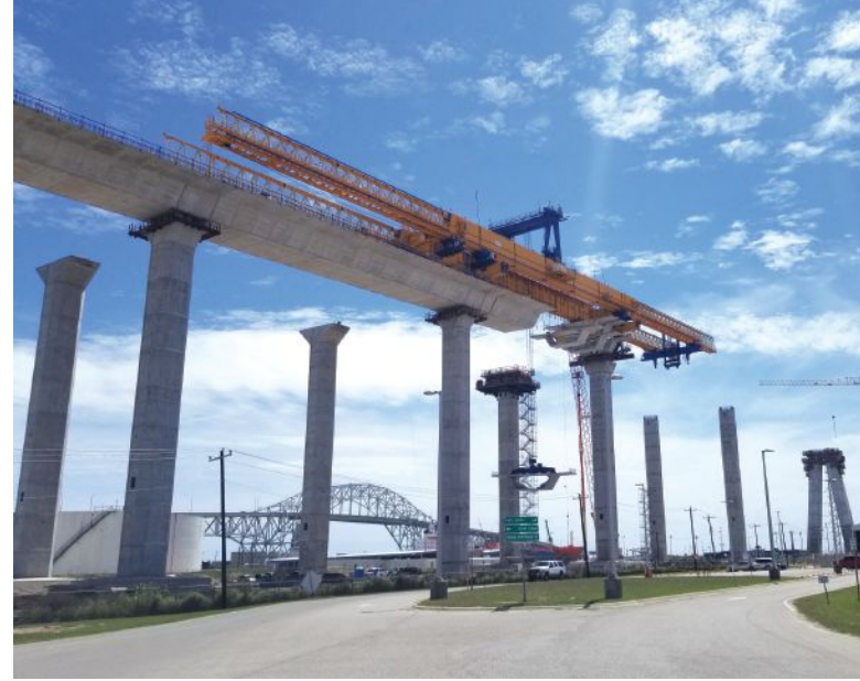
Figure 3. A launching gantry erects an approach span on the Harbor Bridge project in Corpus Christi, Tex. Self-weight of gantries and suspended loads during construction may control the substructure and foundation designs of a bridge. Photo: Flatiron Dragados JV.
