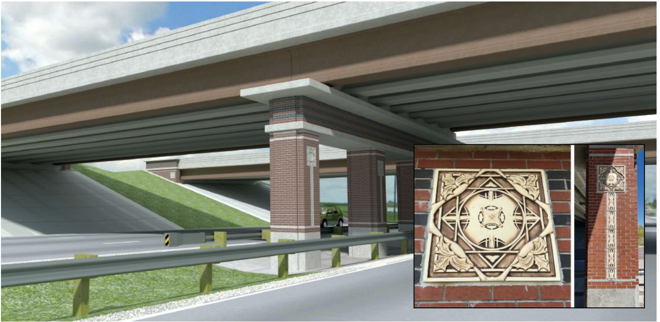
Figure 2. Interstate 80 interchange at Grinnell, Iowa. Thin brick veneer and copings were used to bring historically significant framework and architectural elements to the piers of the structures. Rendering and Photos: Iowa Department of Transportation
