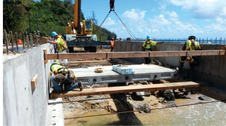
Slow-set epoxy paste adhesive was applied to the joint faces of the precast concrete slabs before erection. The slow-set epoxy was used to ensure that there was adequate time to set and post-tension the slabs. Photo: KSF Inc.
