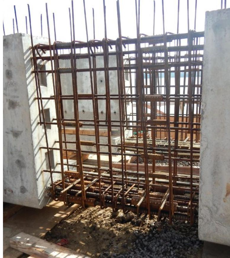
The L-girders were transported to the site in three segments and connected with cast-in-place closure pours on site. Photo: Hawaiian Dredging Construction Company Inc.
