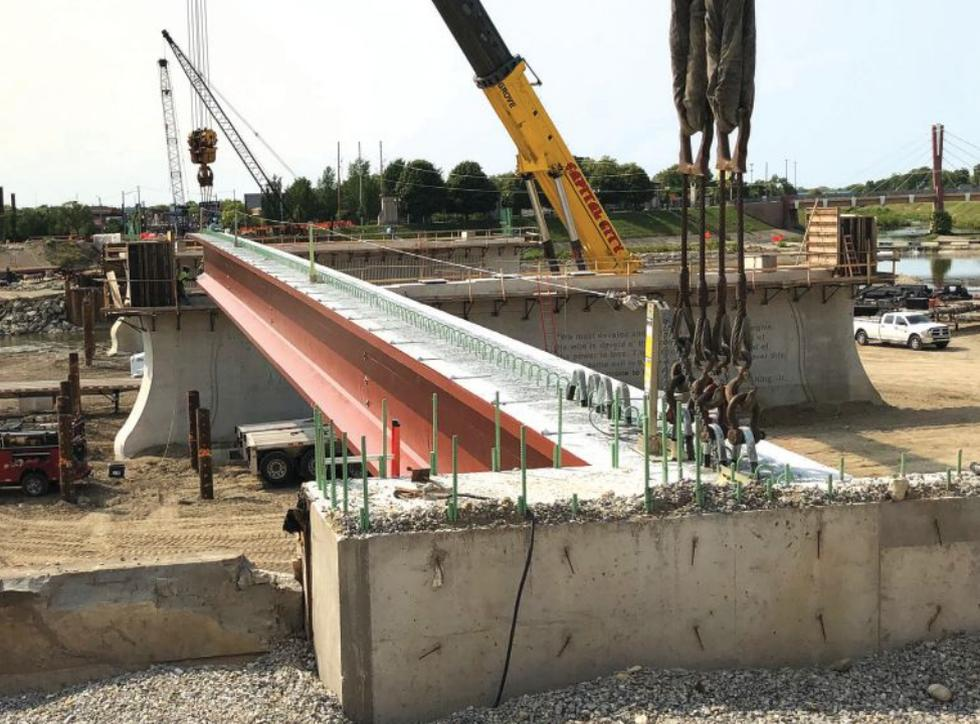
In accordance with Ohio Department of Transportation (ODOT) standards, epoxy-coated reinforcing steel was used in the cast-in-place concrete elements to enhance durability. Glass-fiber-reinforced polymer reinforcement was used in the concrete railings to control cracking and reduce corrosion potential.
