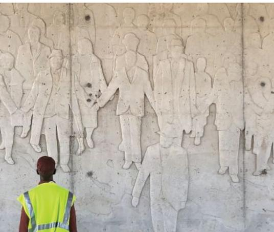
The formliner used to create the image of the 1963 Unity March (top) and the image shortly after form removal (bottom). All Photos: Montgomery County Engineer's Office.
