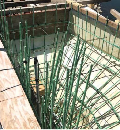
Epoxy-coated reinforcement was placed in the formwork for an overlook support pedestal at a pier. The intricate curvilinear shapes of the piers and overlook supports were made possible by using computer-generated expanded polystyrene foam forms.
