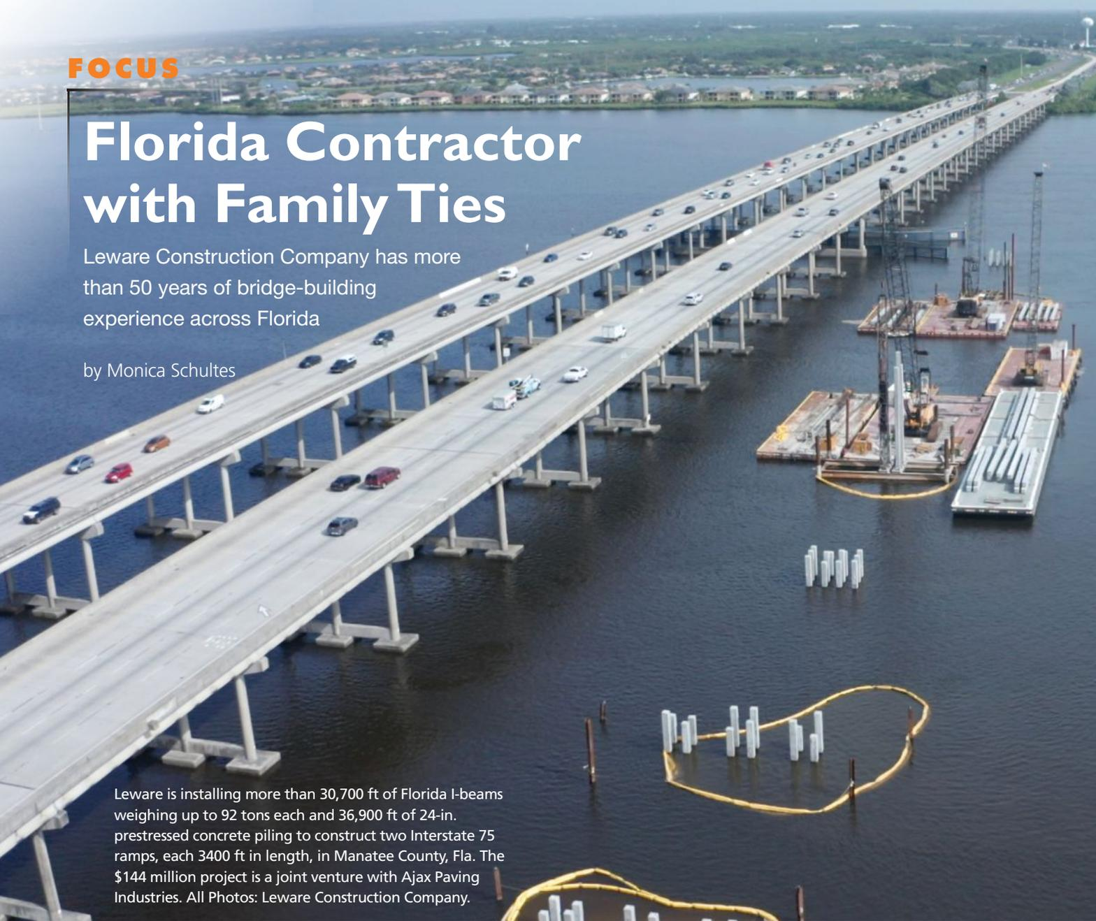
Leware is installing more than 30,700 ft of Florida I-beams weighing up to 92 tons each and 36,900 ft of 24-in. prestressed concrete piling to construct two Interstate 75 ramps, each 3400 ft in length, in Manatee County, Fla. The \$144 million project is a joint venture with Ajax Paving Industries. All Photos: Leware Construction Company.
