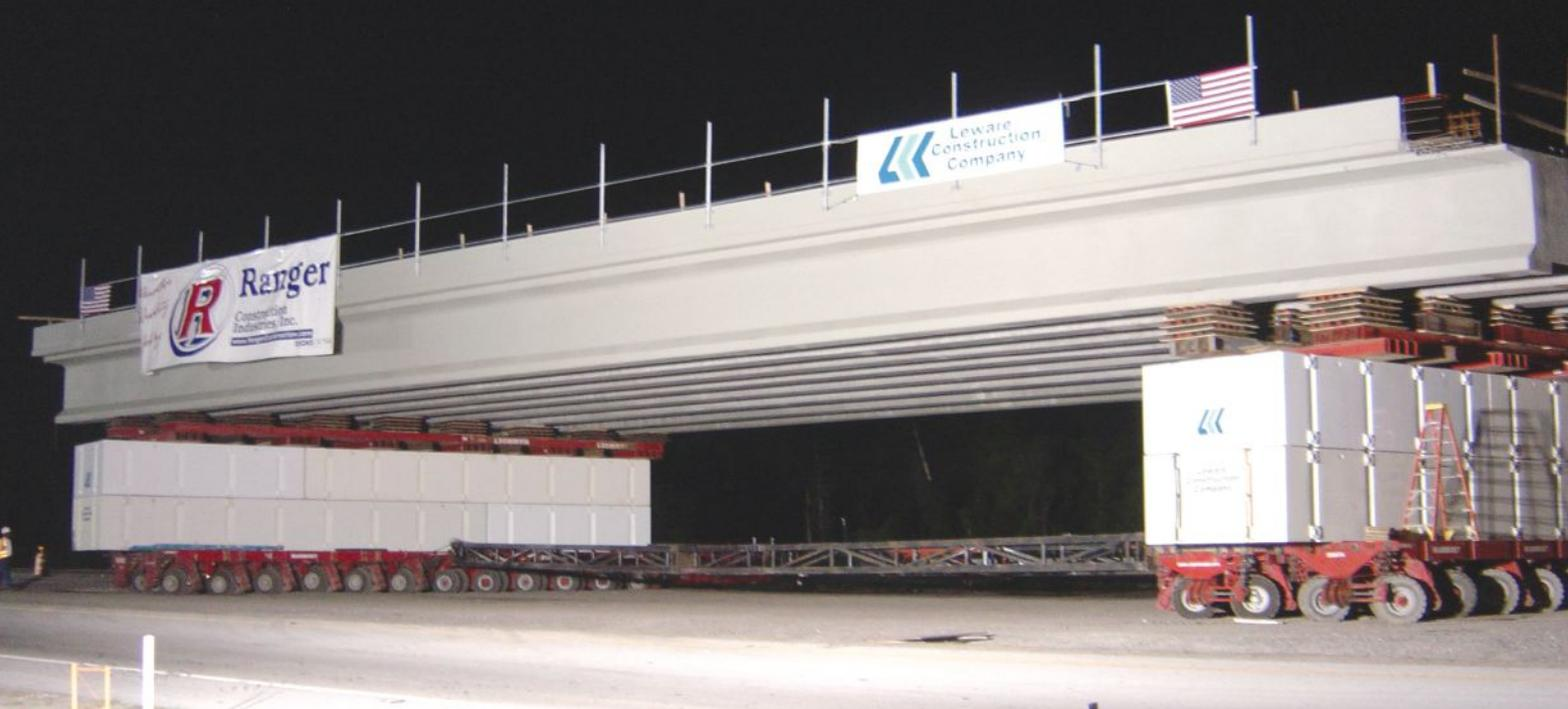
A self-propelled modular transporter (SPMT) was used to move an eight-girder span unit with a concrete deck and railings into position at Graves Road over Interstate 4. Use of the SPMT reduced the road closure from several weeks to two nights.
