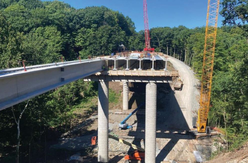
Several of the nearly 8-ft-deep prestressed concrete PA bulb-tee beams were erected by early August 2022. The historic Frick Park Gatehouse is barely visible at the far left corner of the bridge. Photo: HDR Inc.
