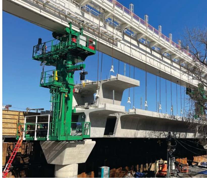
Erection of a precast concrete segment. Photo: Walsh-Fluor Design-Build Team.
