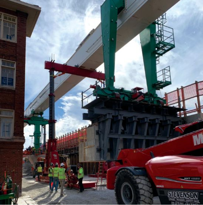
The launching girder assembly. Photo: Walsh-Fluor Design-Build Team.
