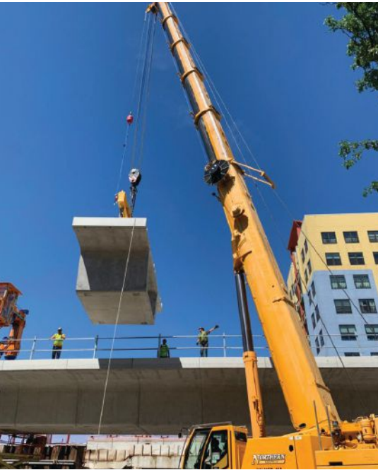
A precast concrete segment is hoisted from a haul truck on the street onto a completed viaduct span before being moved into position by a segment transporter. Photo: Walsh-Fluor Design-Build Team.
