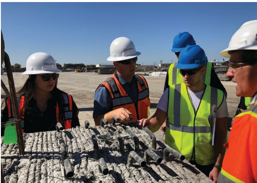
A precaster's chief engineer explains prestressed concrete girder details to students during a tour of a precast concrete plant. Photo: Eric Matsumoto.
