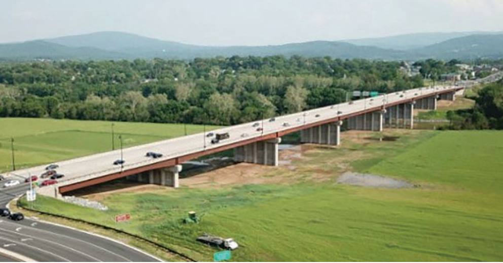
Figure 3. For new construction, continuity and jointless bridge solutions are good options. This bridge has a 1915-ft-long, 100-ft-wide continuous reinforced concrete deck.
