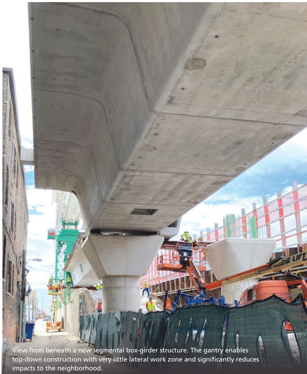
Several precast concrete segments of the second span hang from the gantry as a new segment is hoisted from street level, all while a Chicago Transit Authority Red Line train proceeds unimpeded southbound past the work zone.
