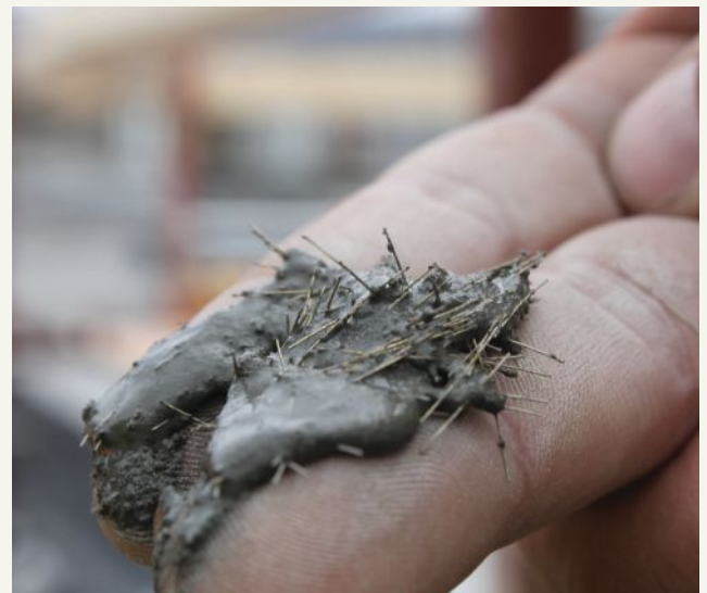
Ultra-high-performance concrete is a high-strength, dense concrete that incorporates random steel fibers and reduces permeability to water, chlorides, and other deleterious materials. It provided a minimum 28-day compressive strength of 21,000 psi for this project. Photo: AECOM.
