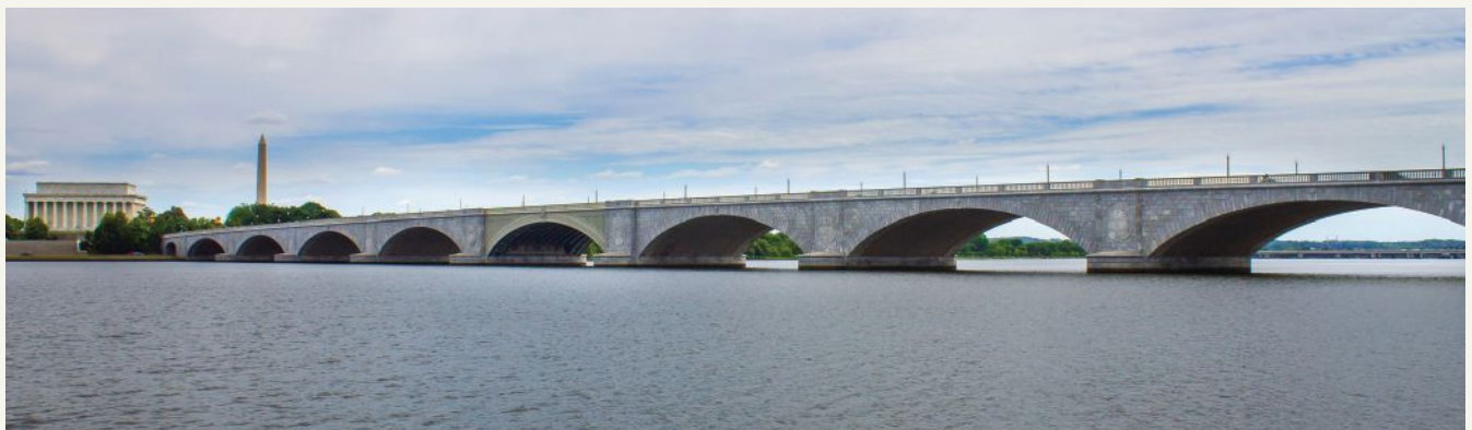
The Arlington Memorial Bridge is a monument to reunification after the Civil War and carries more than 65,000 vehicles daily, linking northern Virginia to Washington, D.C. Photo: AECOM.
