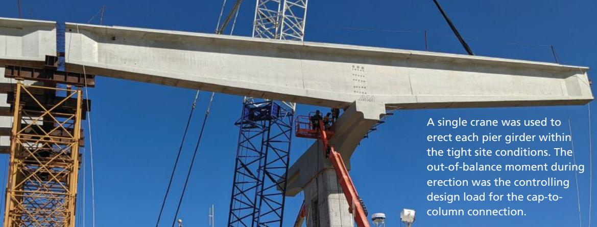
A single crane was used to erect each pier girder within the tight site conditions. The out-of-balance moment during erection was the controlling design load for the cap-to-column connection.
