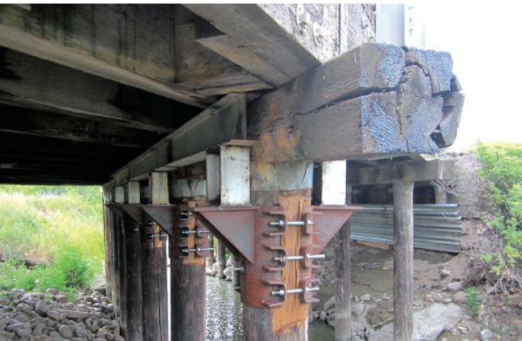
The Clear Creek timber bridge, which had abutment and bank scour and previously repaired timber members, needed replacement. Photos: Montana Department of Transportation.
