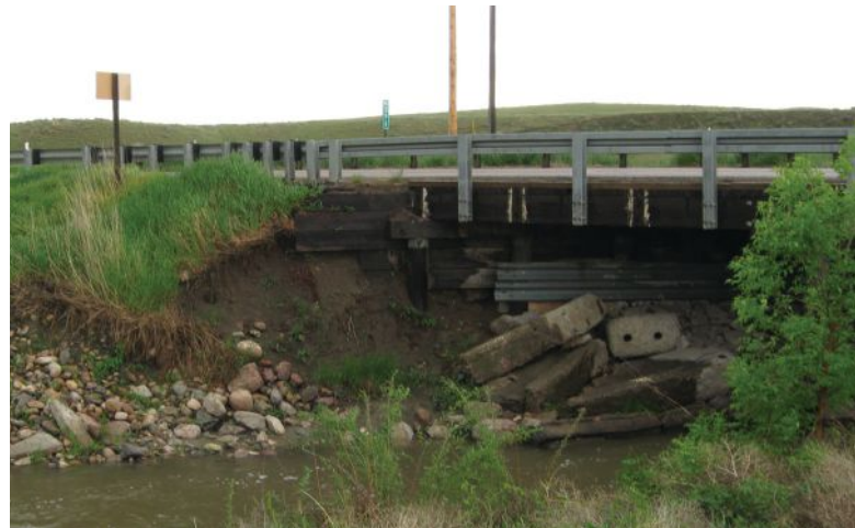
The Clear Creek timber bridge, which had abutment and bank scour and previously repaired timber members, needed replacement. Photos: Montana Department of Transportation.
