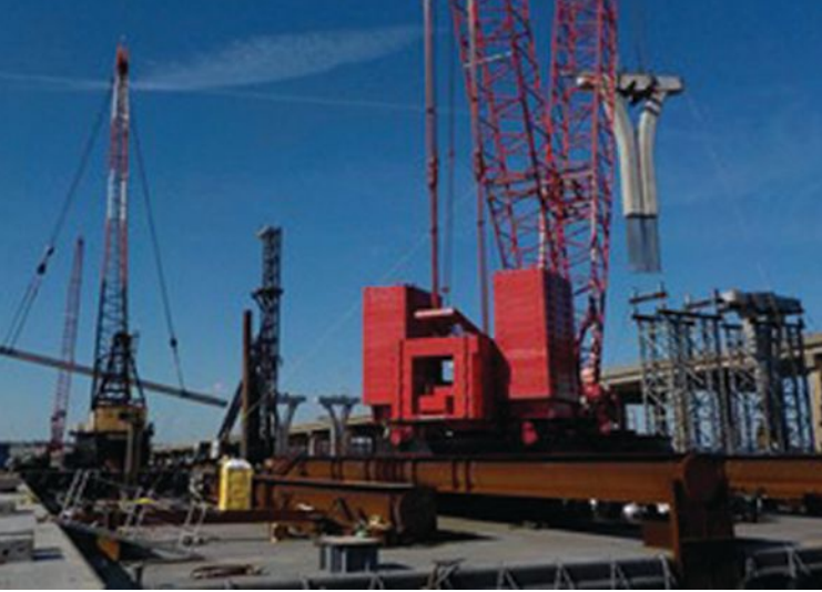
A taller precast concrete V-pier column and cap segment being set on falsework that will support it before a pressure concreted closure pour is placed to connect the unit to the footing. Photo: WSP USA.
