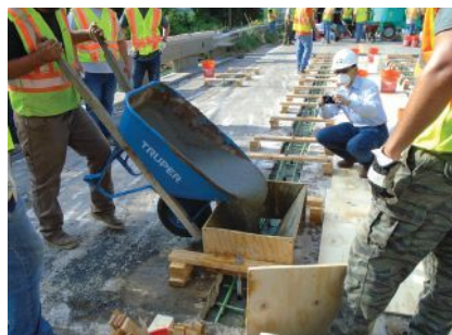
Developed at the University of Michigan, the open-recipe ultra-high-performance concrete (UHPC) was carefully batched in small amounts on site (left) for deck closure pours for the Kilgore Road Bridge Restoration Project in Kenockee, Mich. This demonstration project was one of the earliest field applications of a nonproprietary UHPC in the United States. UHPC is placed in the closure joint after being batched with the light blue mixer visible in the background (center). The protruding all-thread rods visible in the photo on the right support the bottom formwork to prevent leakage during placement of the UHPC in the closure joints. All Photos: Clare County Road Commission.
