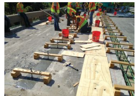
Developed at the University of Michigan, the open-recipe ultra-high-performance concrete (UHPC) was carefully batched in small amounts on site (left) for deck closure pours for the Kilgore Road Bridge Restoration Project in Kenockee, Mich. This demonstration project was one of the earliest field applications of a nonproprietary UHPC in the United States. UHPC is placed in the closure joint after being batched with the light blue mixer visible in the background (center). The protruding all-thread rods visible in the photo on the right support the bottom formwork to prevent leakage during placement of the UHPC in the closure joints. All Photos: Clare County Road Commission.
