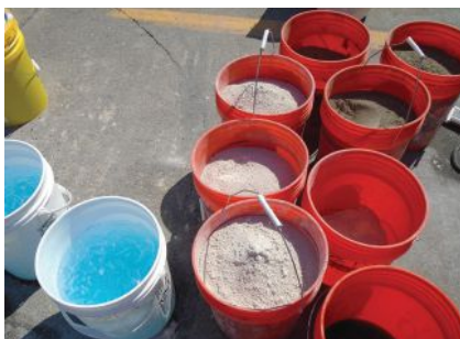
Developed at the University of Michigan, the open-recipe ultra-high-performance concrete (UHPC) was carefully batched in small amounts on site (left) for deck closure pours for the Kilgore Road Bridge Restoration Project in Kenockee, Mich. This demonstration project was one of the earliest field applications of a nonproprietary UHPC in the United States. UHPC is placed in the closure joint after being batched with the light blue mixer visible in the background (center). The protruding all-thread rods visible in the photo on the right support the bottom formwork to prevent leakage during placement of the UHPC in the closure joints. All Photos: Clare County Road Commission.
