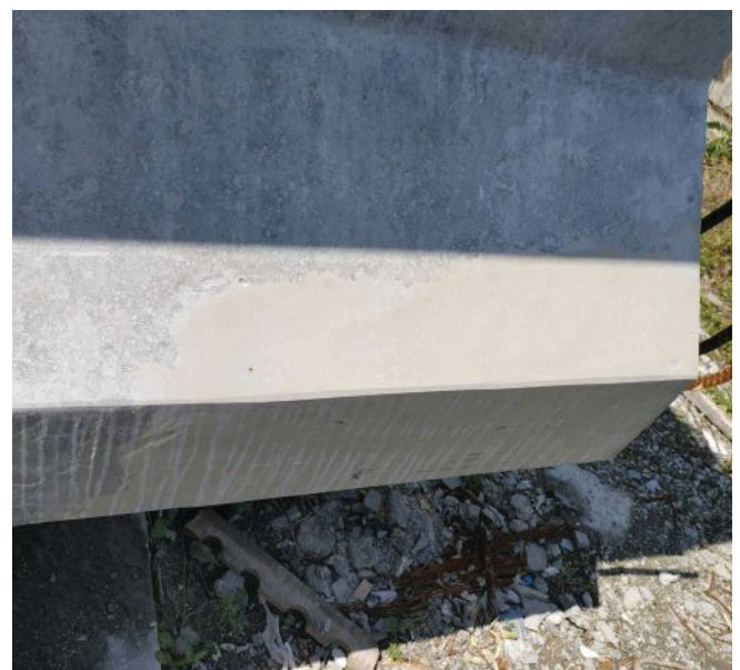
Void in the bottom flange at the end of a girder observed after form removal (left). Completed repair of void after finishing (right). A high-modulus, two-component structural epoxy adhesive that was mixed with oven-dried sand was used for the repair, which was similar to North Carolina Department of Transportation Standard Repair Procedure, but on a larger scale. All Photos: North Carolina Department of Transportation.
