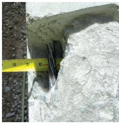
Photos of the preparation and repair of a defect at the corner of the bottom flange of a prestressed concrete girder. The left photo is a close-up of the area prepared for repair by removing unsound concrete from the void area and squaring the edges. The center photo is an overhead view of the same area to be repaired where concrete has been chipped out behind the strand. The right photo shows the completed repair. An on-site North Carolina Department of Transportation (NCDOT) inspector documents the defect, is present during the repair, and, if satisfied, approves the repair. This defect is similar to one of the NCDOT Standard Repair Procedures, but it is deeper than the limit so the Materials and Tests Unit inspector needs to document the defect. That documentation, along with the producer's detailed repair procedure, is then submitted as a nonconformance report to the Structures Management Unit for review and approval.
