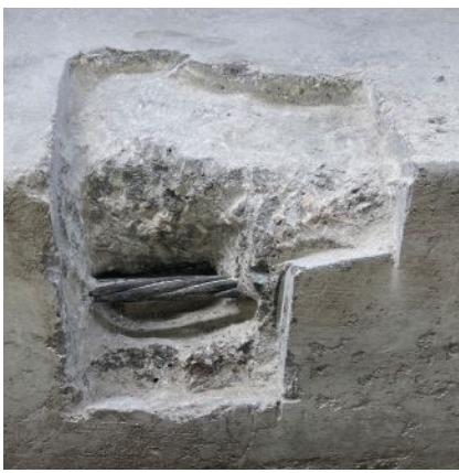
Photos of the preparation and repair of a defect at the corner of the bottom flange of a prestressed concrete girder. The left photo is a close-up of the area prepared for repair by removing unsound concrete from the void area and squaring the edges. The center photo is an overhead view of the same area to be repaired where concrete has been chipped out behind the strand. The right photo shows the completed repair. An on-site North Carolina Department of Transportation (NCDOT) inspector documents the defect, is present during the repair, and, if satisfied, approves the repair. This defect is similar to one of the NCDOT Standard Repair Procedures, but it is deeper than the limit so the Materials and Tests Unit inspector needs to document the defect. That documentation, along with the producer's detailed repair procedure, is then submitted as a nonconformance report to the Structures Management Unit for review and approval.
