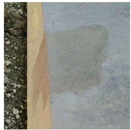
Photos of the preparation and repair of a defect at the corner of the bottom flange of a prestressed concrete girder. The left photo is a close-up of the area prepared for repair by removing unsound concrete from the void area and squaring the edges. The center photo is an overhead view of the same area to be repaired where concrete has been chipped out behind the strand. The right photo shows the completed repair. An on-site North Carolina Department of Transportation (NCDOT) inspector documents the defect, is present during the repair, and, if satisfied, approves the repair. This defect is similar to one of the NCDOT Standard Repair Procedures, but it is deeper than the limit so the Materials and Tests Unit inspector needs to document the defect. That documentation, along with the producer's detailed repair procedure, is then submitted as a nonconformance report to the Structures Management Unit for review and approval.
