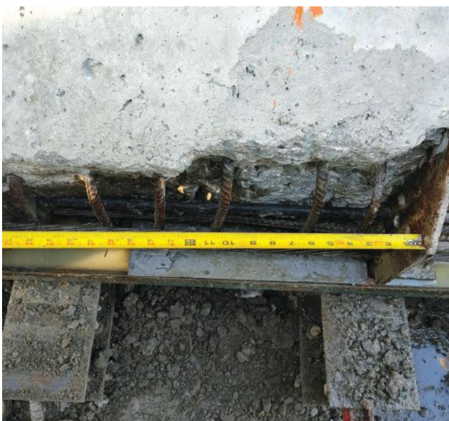
Void in the bottom flange at the end of a girder observed after form removal (left). Completed repair of void after finishing (right). A high-modulus, two-component structural epoxy adhesive that was mixed with oven-dried sand was used for the repair, which was similar to North Carolina Department of Transportation Standard Repair Procedure, but on a larger scale. All Photos: North Carolina Department of Transportation.
