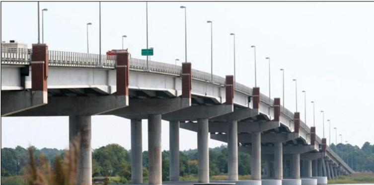
The Virginia Route 33 Bridge over the Mattaponi River has post-tensioned lightweight concrete spliced girders with a lightweight concrete deck to achieve two units with spans of 200-240-240-200 ft. Photo: Kenneth S. Harmon
