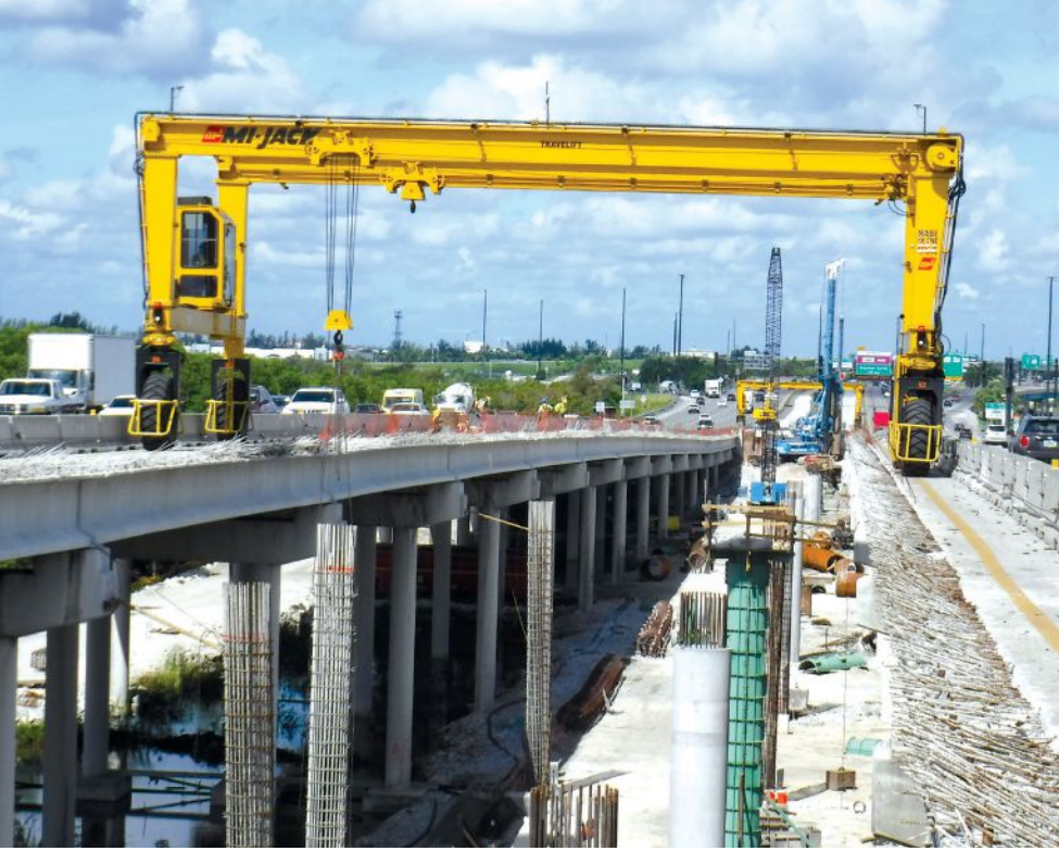
Figure 2. The rubber-tired gantry crane requires just 5 ft of aisle way on either side to handle loads.
