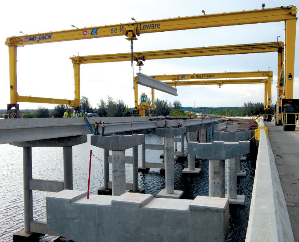
Figure 4. Expanding the lanes of an interstate bridge that services thousands of cars per day poses right-of-way and traffic flow challenges. Gantry cranes can provide a practical and economical solution where access is limited.
