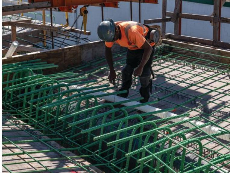
All reinforcement in the box-girder superstructure is epoxy coated for durability. Although deicing salts will not be used on the light rail structure, there is potential for chloride exposure given its proximity to adjacent roadways. The worker is installing a longitudinal post-tensioning duct in the last cantilever segment adjacent to a closure pour location.
