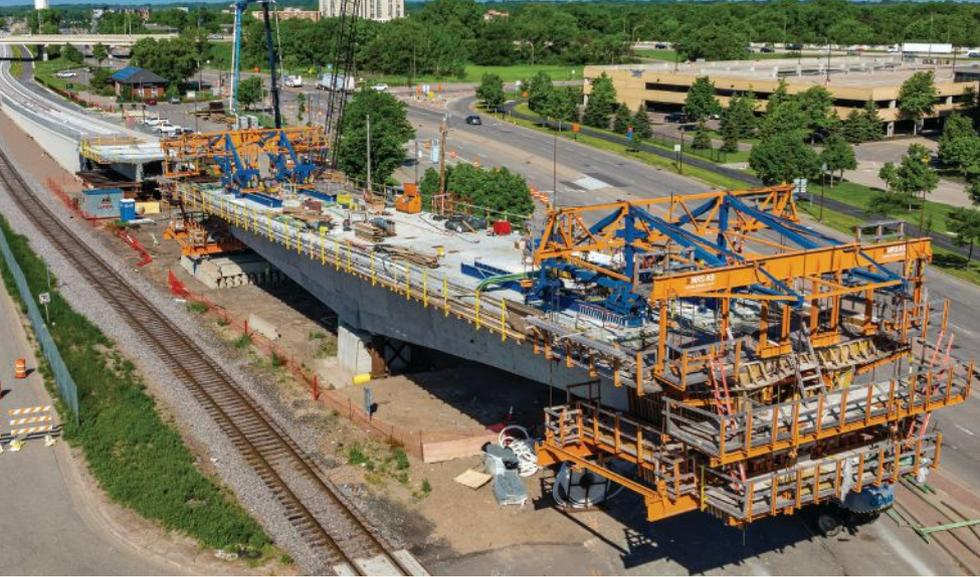
Construction of both cantilevers at the first pier uses a form traveler at each end. A temporary support is visible at the pier, and the portion of the first span that was cast on falsework is visible in the background. The bridge is close to an active freight rail line, which, once relocated, will be within 15 ft of the new structure in some locations.
