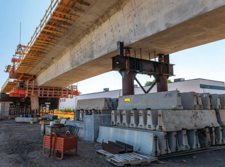
A ballasted, temporary stability prop located under the fourth segment on the longer side of the cantilever is used to provide rotational stability for the box-girder span and resist uplift during balanced-cantilever construction. In the background of the photo, the portion of the span connecting to the abutment is being cast on falsework.
