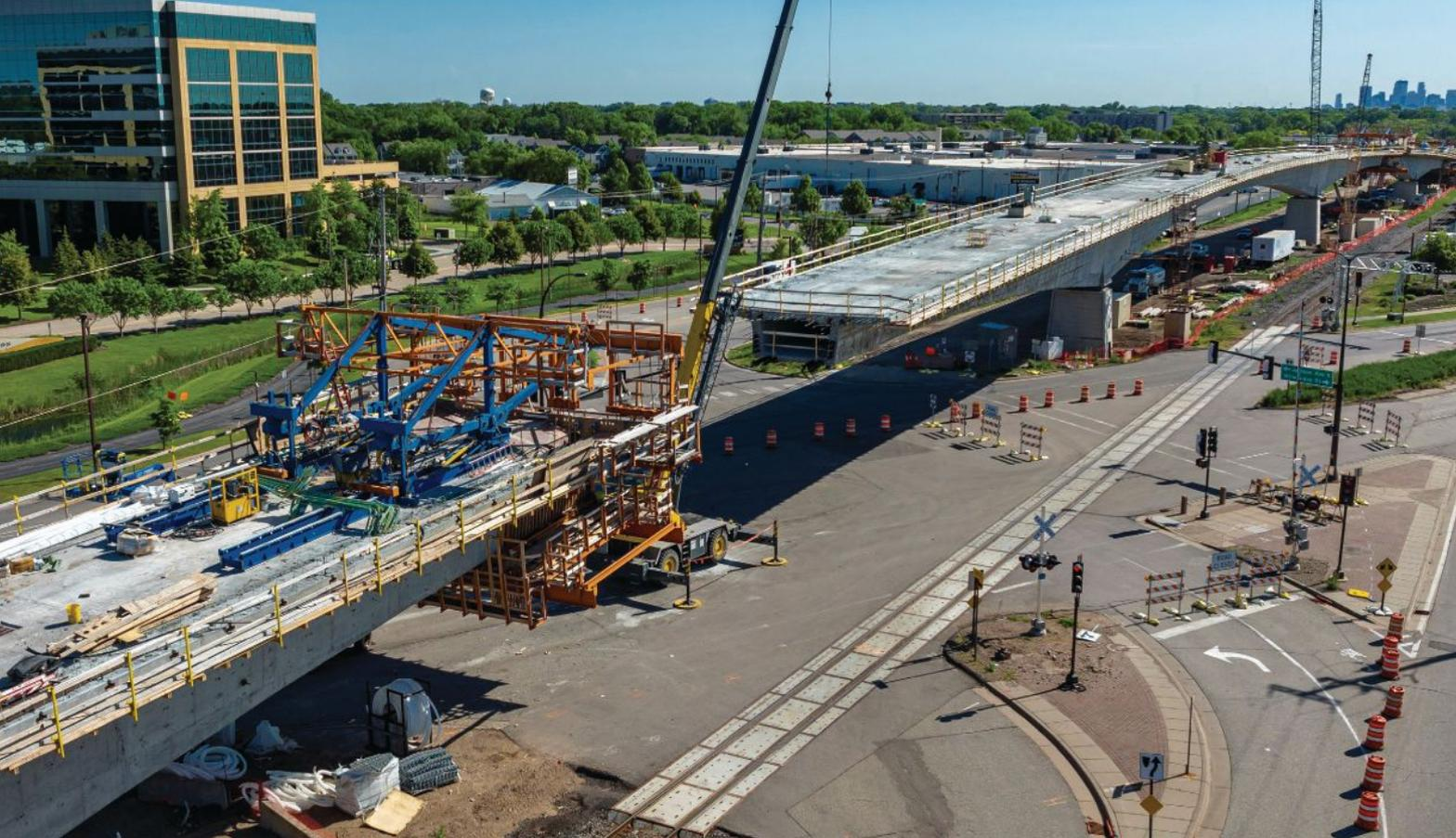
Balanced-cantilever construction with form travelers nears completion. The final closure pour of the 1608-ft-long, post-tensioned, cast-in-place concrete segmental box-girder bridge will be at this location in span 2 over Excelsior Boulevard, after the cantilever is completed.
