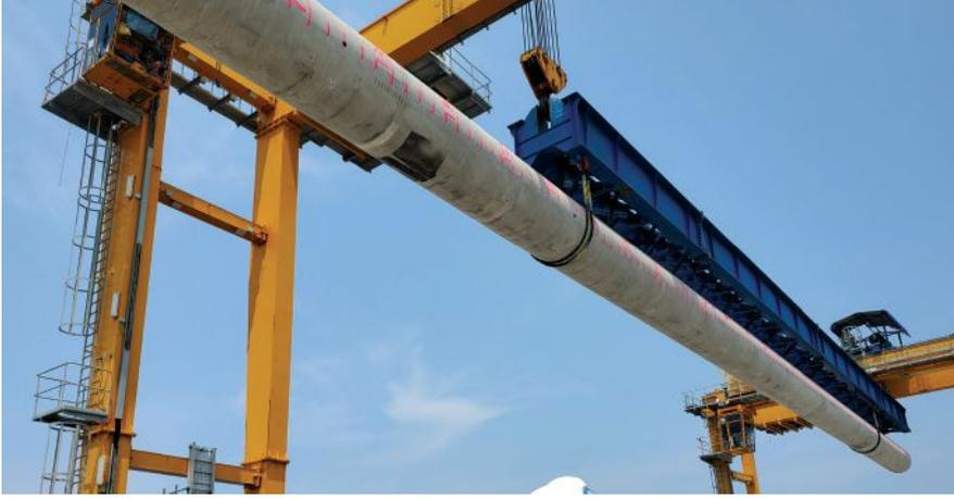
An overhead gantry working from an advancing rail system parallel to the outside edge of the bridge after it lifts a prestressed concrete cylinder pile from a vehicle on the completed portion of the bridge and moves it ahead to be installed. The 54-in.-diameter prestressed concrete cylinder piles, with lengths up to 165 ft, were used for the foundations of the bridge's main spans.
