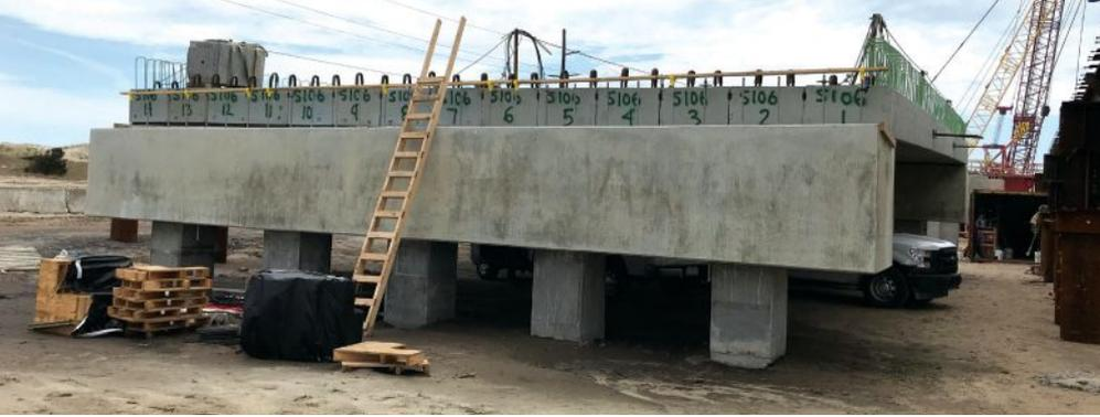
Approach spans used 24-in.-deep prestressed concrete voided slabs on bents with 30-in.-square prestressed concrete piles.
