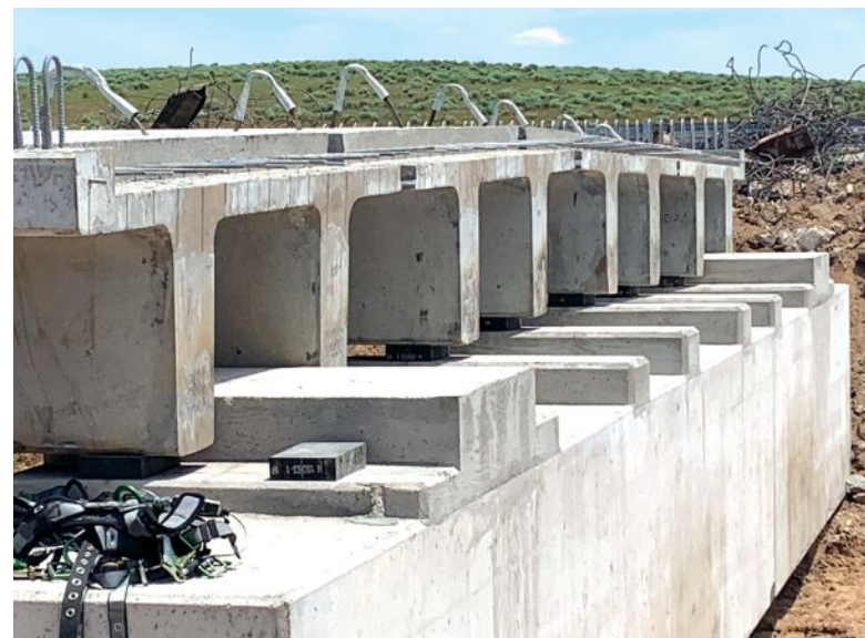
The 2¾-in.-thick elastomeric bearing pads are beveled 0.25 in. to match the 2% roadway cross slope and allow level bearing seats.
