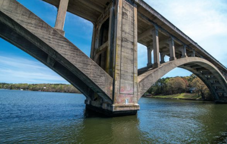
The original open-spandrel arch bridge had a 20-ft-wide deck. Photo: AECOM, courtesy of Byrd's Eye View.
