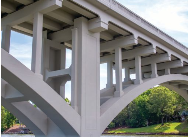
The new superstructure of the rehabilitated bridge has a 36-ft-wide road surface. Establishing continuity of the prestressed concrete box beams from pier to pier before placing the concrete deck mitigated loadings on the arch ribs. Photo: AECOM.
