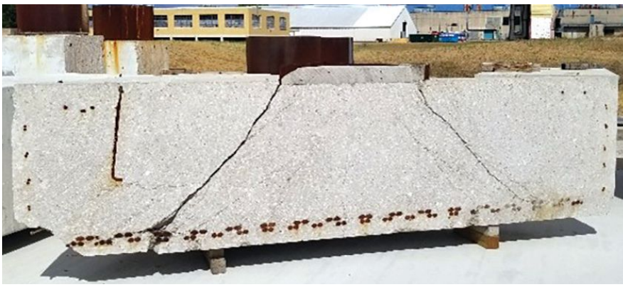
The Concrete Bridge Engineering Institute (CBEI) has a collection of concrete bridge components that will be used to help participants compare theoretical behavior to actual test results, and predict and evaluate cracks in concrete. Photo: CBEI.
