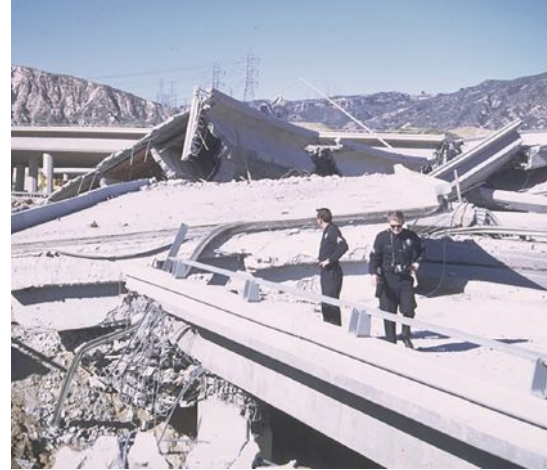
Figure 1. Bridge damage from the 1971 San Fernando earthquake. All Photos and Figures: California Department of Transportation.
