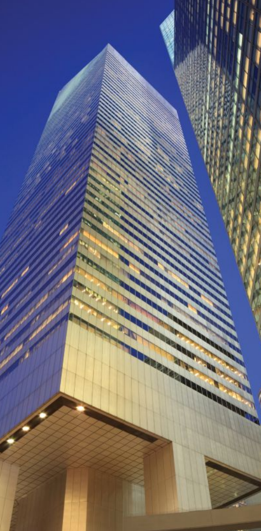
Figure 2. A single phone call started a chain of events that potentially saved the Citicorp Center in New York City from collapse. A culture of empowerment can bring the code of ethics to life and protect the health, safety, and welfare of the public. Photo: Structural Technologies.
