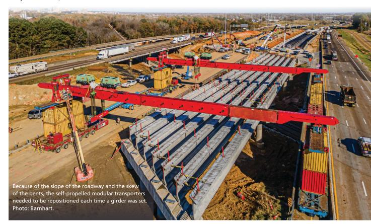
$\mathbf{K}^{\text{ey}}$  Constructors' megaproject on Interstate 20 (I-20) resembles central Houston, Tex., more than the south side of Jackson, Miss., given the number of bridges, service roads, and on-ramps in the vicinity. The contractor is threading a needle as it replaces a deteriorated section of the I-20 eastbound bridge with a larger 14-span bridge at the confluence of I-20 with Interstate 55 (I-55) and U.S. Highway 51 (U.S. 51).
