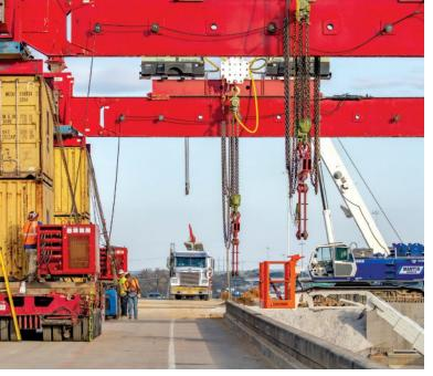
Engineers analyzed the existing bridges to ensure that they had sufficient structural capacity to support the self-propelled modular transporters and the massive girders during the erection operation. Photo: Key Constructors.
