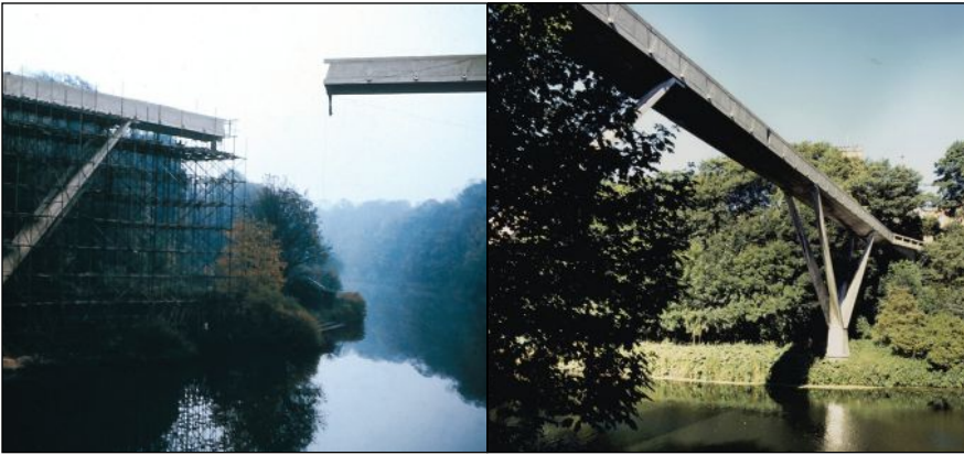
Ove Arup’s design of the Kingsgate Bridge, Durham, England, in 1963 was prescient of our current mode of accelerated bridge construction. The two cantilever sections of this pedestrian bridge were swung out and connected in less than an hour. The Kingsgate Bridge was the last project that Ove Arup designed and epitomizes his philosophy of total design integrating engineering and architecture. Photo: Arup.
