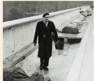
Ove Arup on the Kingsgate Bridge during construction. Photo: Arup.
