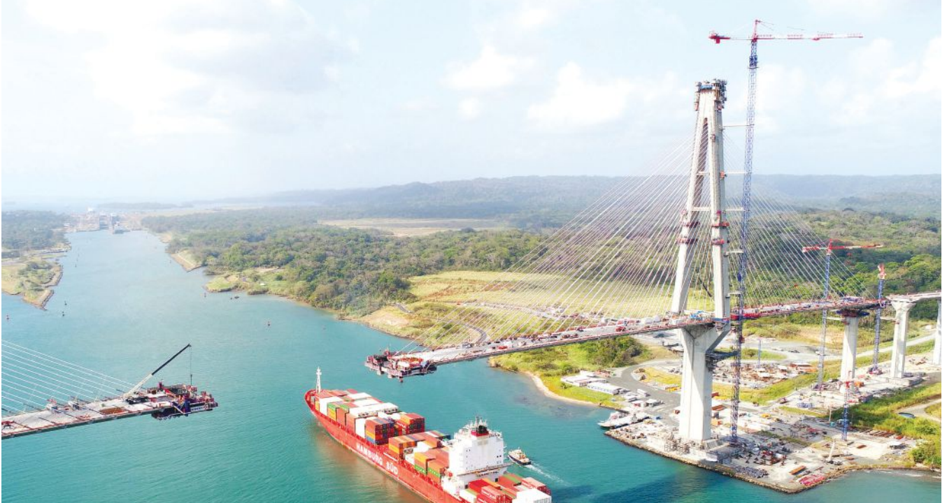
The now completed 1.91-mile-long Atlantic Bridge across the Panama Canal has a 1740 ft main span, which was built using the balanced-cantilever method with traveling forms. The concrete superstructure for the cable-stayed spans consists of longitudinal concrete boxes connected with transverse diaphragms. The deck is supported by two planes of stay cables anchored along the edges. During bridge construction, the Panama Canal could not be closed to shipping or used for construction access. Photo: VINCI Photo Library.
