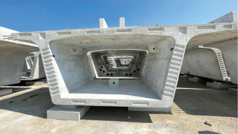
Precast concrete segments for the Red-Purple Modernization project in Chicago, Ill. Although this is the first use of precast concrete segmental construction for the Chicago Transit Authority, the technology has been widely used around the world since Jean M. Muller, the famous French bridge designer and inventor, transformed segmental concrete bridge design. Several bridge engineers at International Bridge Technologies worked directly with Muller. Photo: SYSTRA-IBT.
